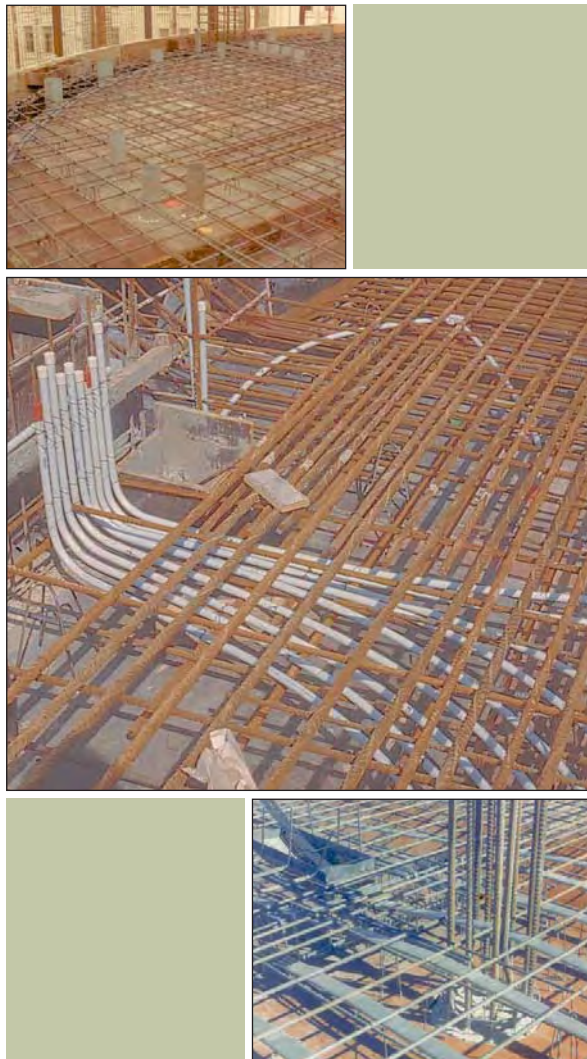
FIGURE 3: Services and penetrations through slabs
