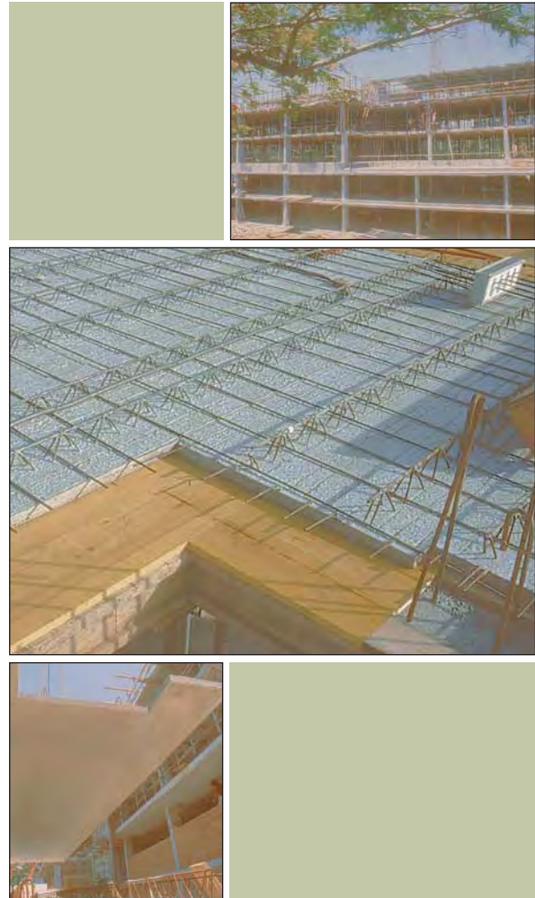
FIGURE 16: Permanent formwork or soffit slabs
