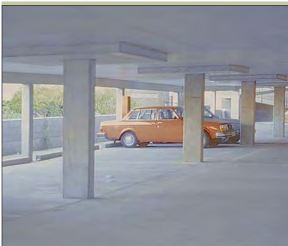
FIGURE 9: Flat slab floor system
