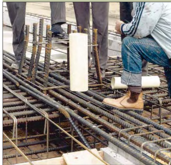
FIGURE 7: Mock-up of complicated reinforcement details
