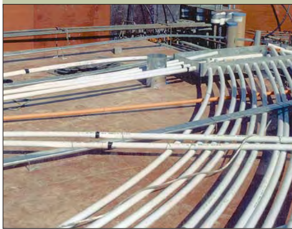
FIGURE 2: Cables placed within a slab
