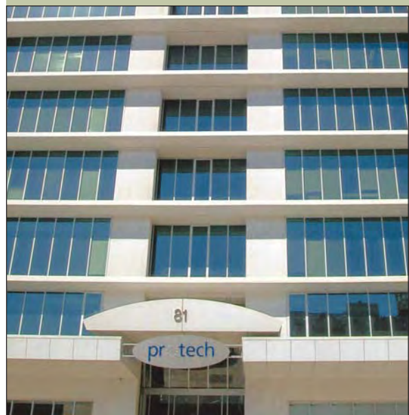
FIGURE 5: Cantilevered floor slabs
