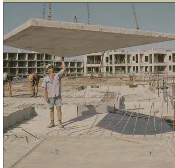
FIGURE 18: Lifting of solid slab unit
