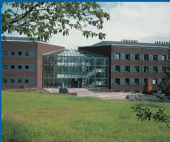
Left: University College Cork, flat slab and waffle slab stressed with unbonded tendons
