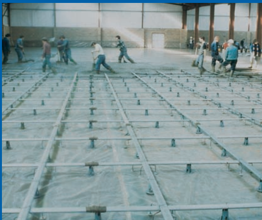
Post-tensioned warehouse ground slab
