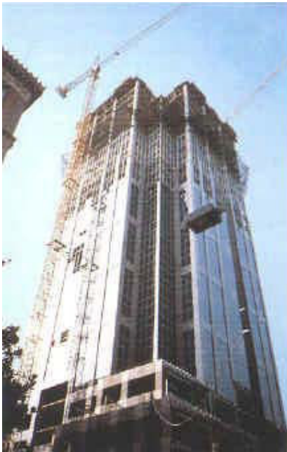
Fig. 2.1: Typical High-Rise Building under Construction
