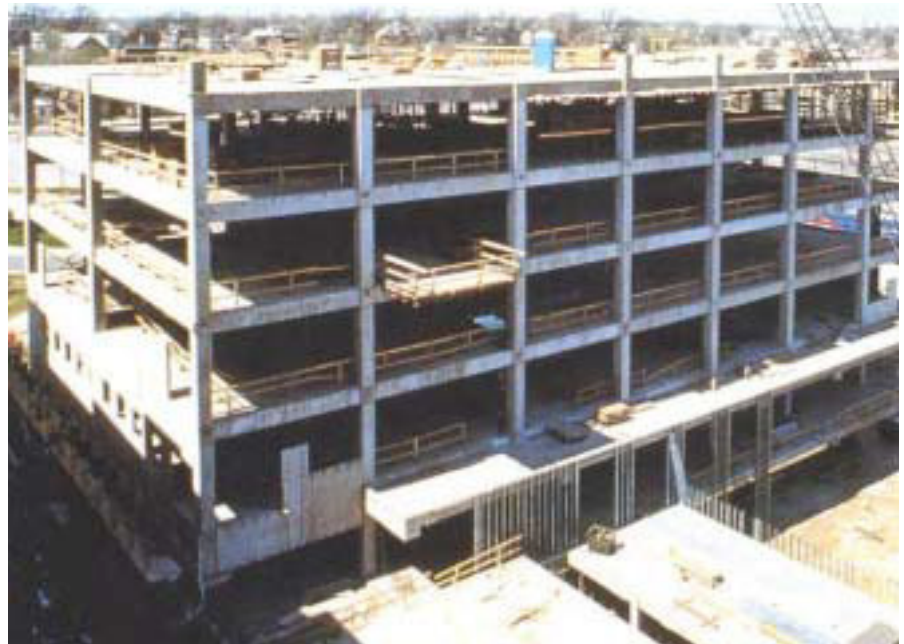
Fig. 2.2: Typical Low-Rise Building under construction
